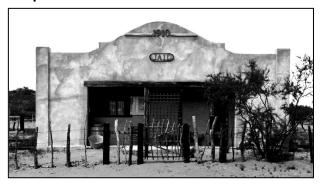
Completed in April of 1910, the jail was built entirely of reinforced concrete at a cost of \$1,778. It originally had two cells, and replaced a temporary wooden jail which had a tin roof. The concrete building originally had a single steel door in the middle, which opened into an interior hallway. This hallway is now the open-air "porch" in the front of the building. Each cell had a barred interior door, and barred windows on the side and back.
